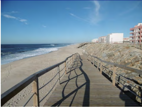
a) Urban waterfront and existing rocky revetment
